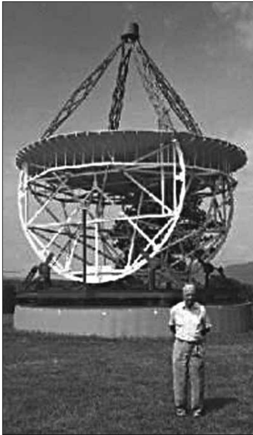
Fig 1.7: Grote Reber standing next to his preserved antenna shortly before his death. In this picture, the dish has been adapted to be rotatable on a turntable mount, so making it a true Az-El mount
